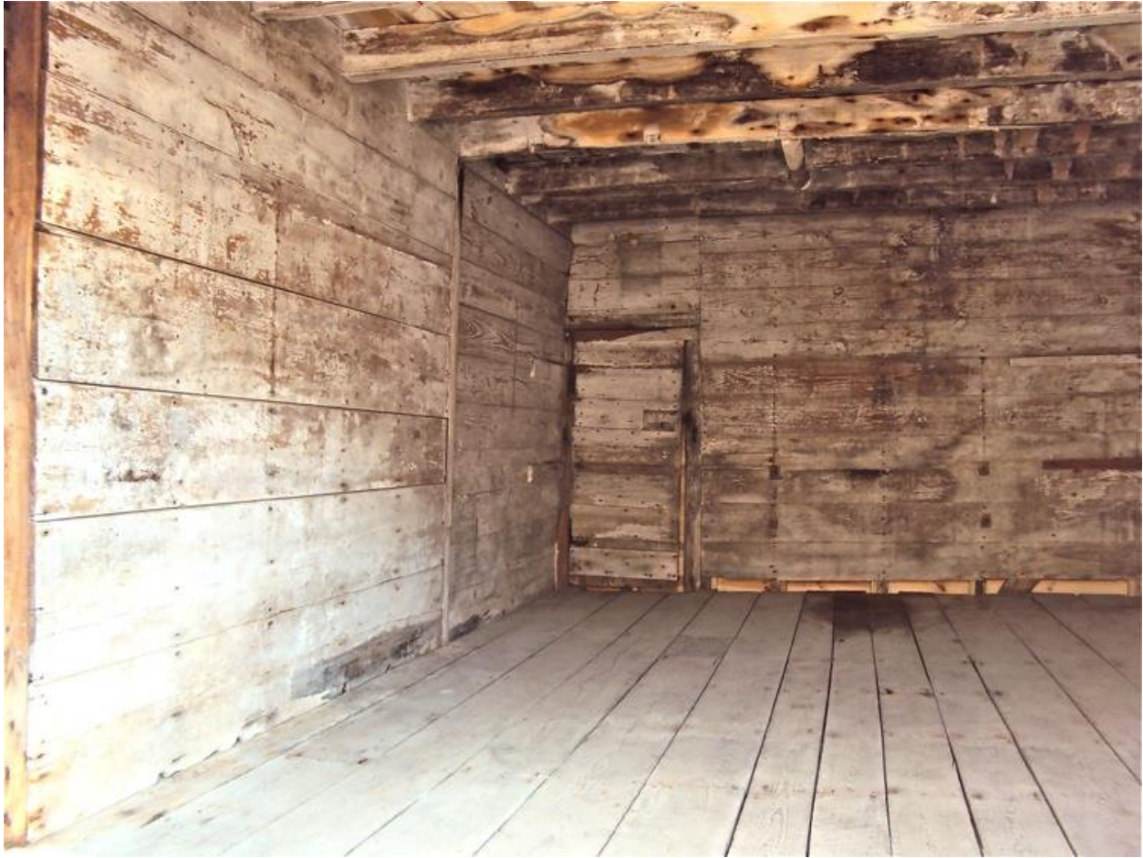
Original back (now west) interior wall of old store
