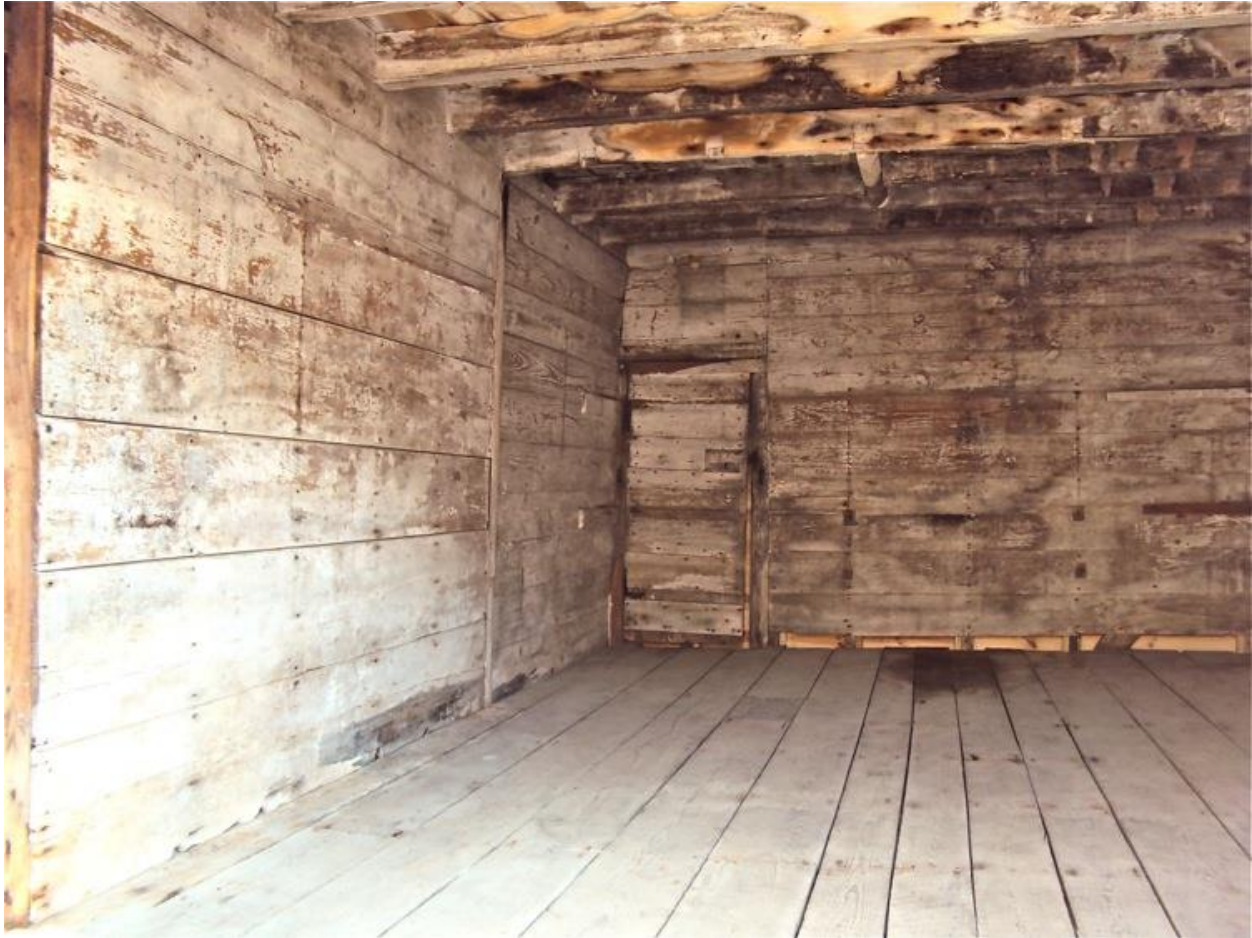
Original front (now east) interior wall of old store
