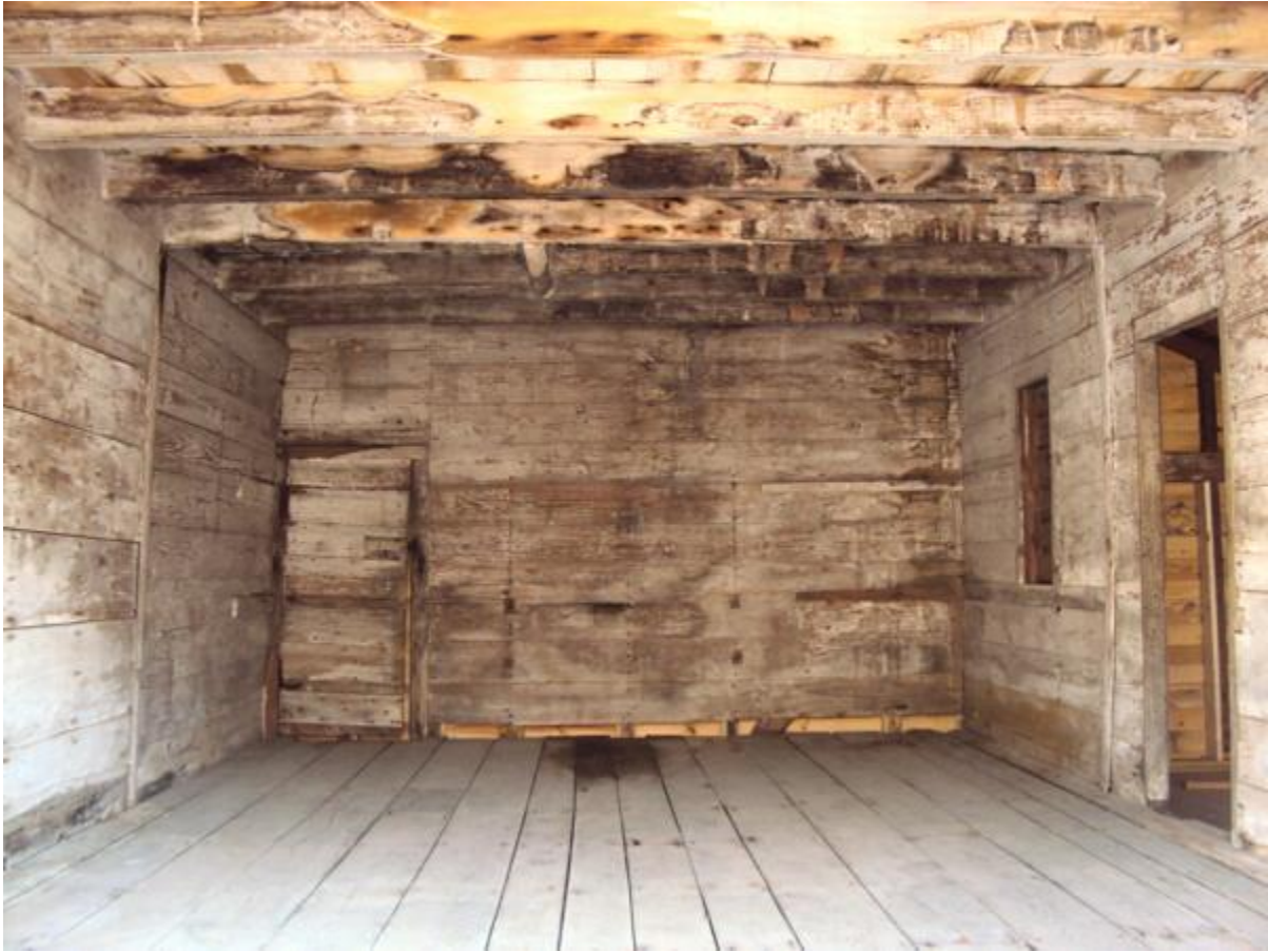
Original south (now north) interior wall of old store
